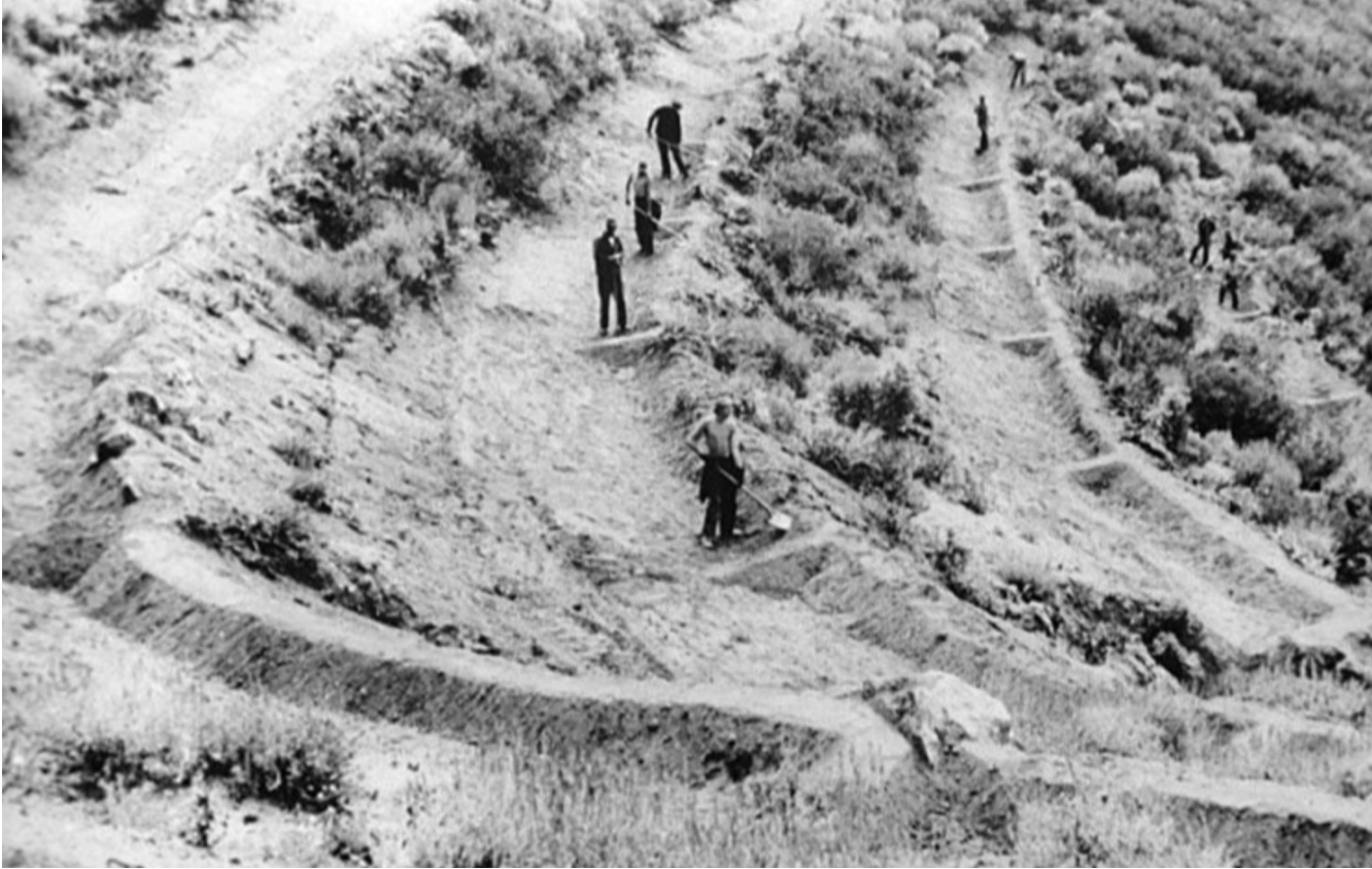
Civilian Conservation Corps building contour-terraces in Utah
