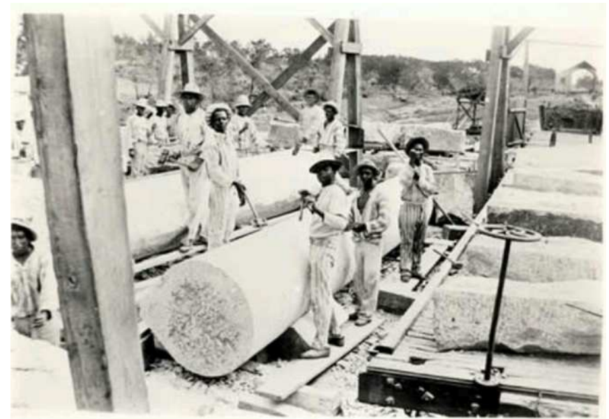
Granite Mountain workers loading cut granite blocks and columns onto a flatbed train car.
